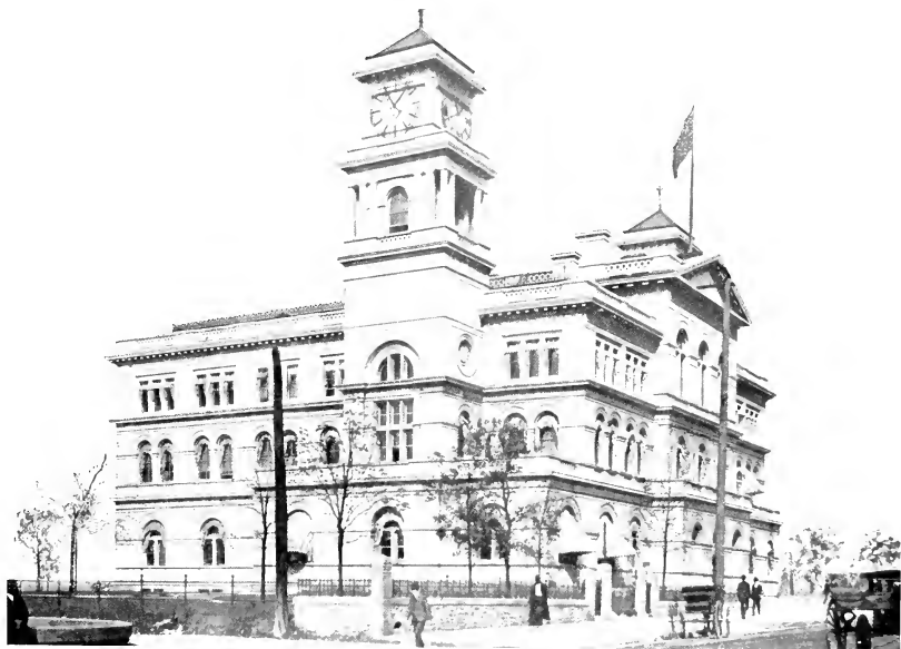
CUSTOM HOUSE AND POST OFFICE
